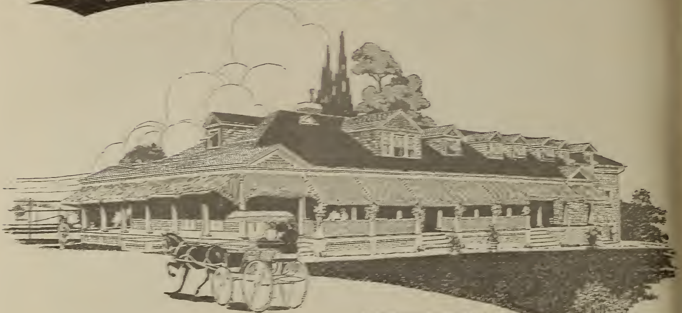
FAIRFIELD COUNTY COUNTRY CLUB GREENWICH, CONN.
