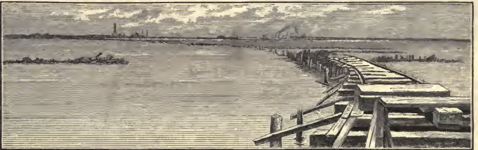
PORT EADS FROM WEST JETTY CONCRETE WHARF.
