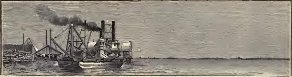
WORK-SHOPS, DERRICK, DREDGE AND JETTY TUG, PORT EADS, LOOKING DOWN THE PASS.
