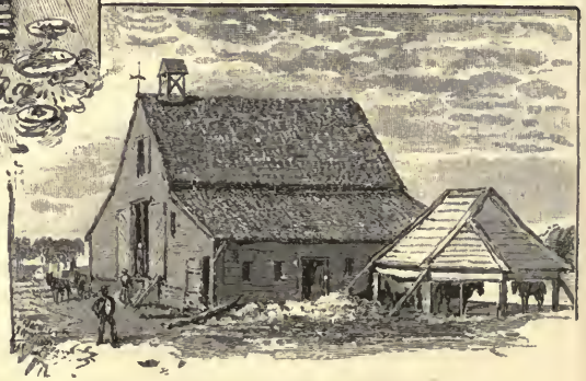
EXTERIOR OF FACTORY.
