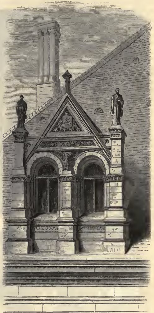
DORMER, COURT SIDE.
