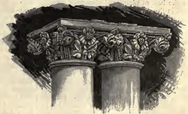
CAPS TO COLUMNS UNDER REPORTERS' GALLERY.
