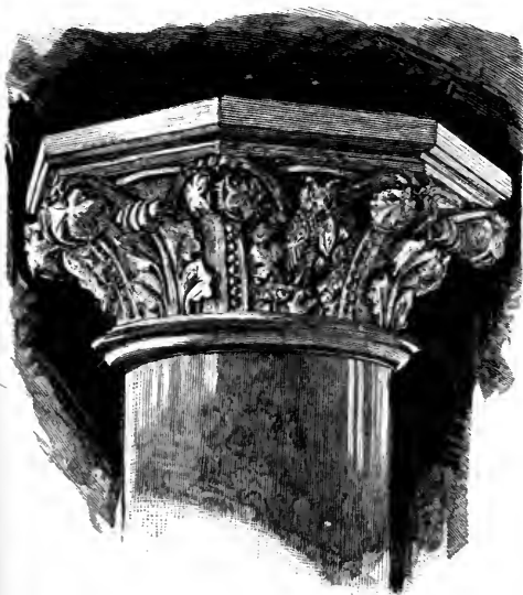
CAP OF LARGE COLUMN, ASSEMBLY ROOM.
