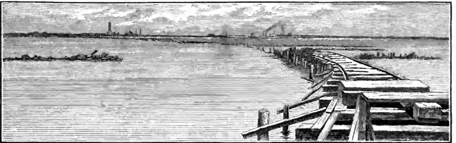
PORT EADS FROM WEST JETTY CONCRETE WHARF.
