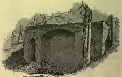
ENTRANCE TO TUNNEL.
