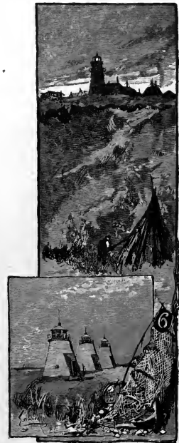
HIGHLAND LIGHT, NORTH TRURO, AND NAUSETT LIGHT, EASTHAM.
