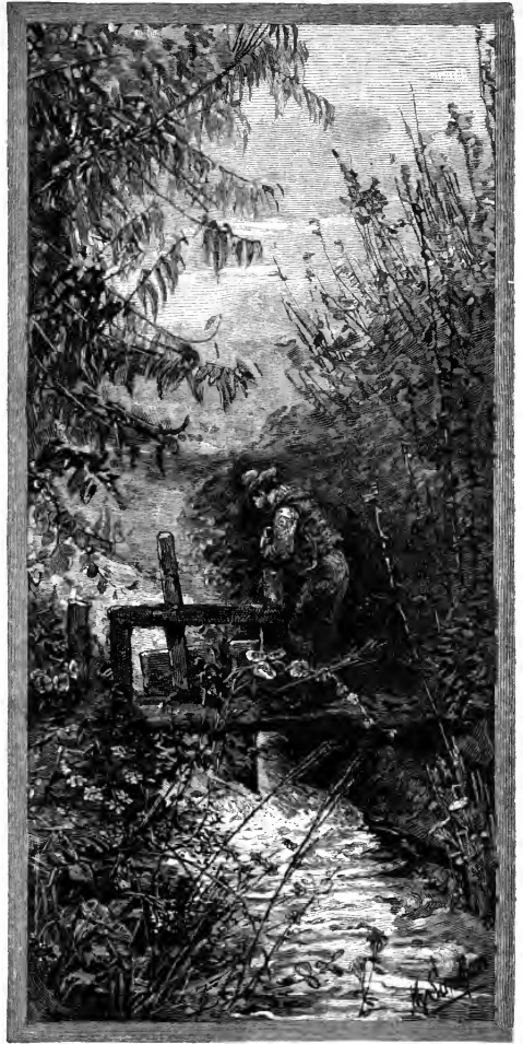
HEAD GATE ON IRRIGATING DITCH.
