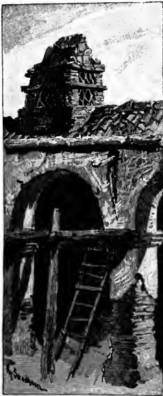
KITCHEN CHIMNEY, SAN JUAN.
