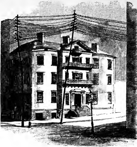
HOUSE CORNER OF BRIDGE AND STATE STREETS.
