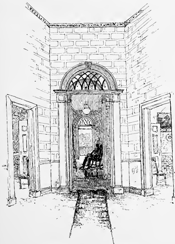
HALLWAY OF THE SPEED HOMESTEAD.
