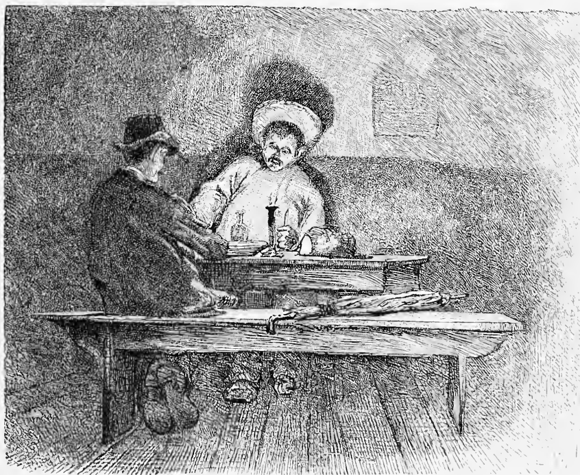
AN INTERIOR AT BIOGE.
