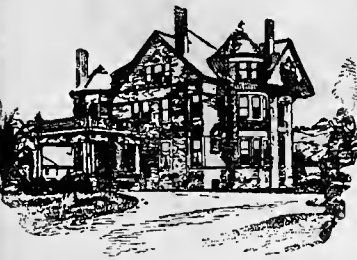
Residence of Capt. J. C. AINSWORTH, Oakland, Cal. Heated by Bolton Heater.
