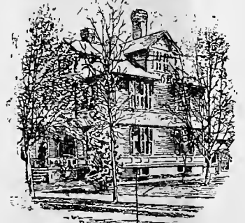
Residence of H. L. NILES, Esq., Springfield, Mass. Heated by Bolton Heater.
