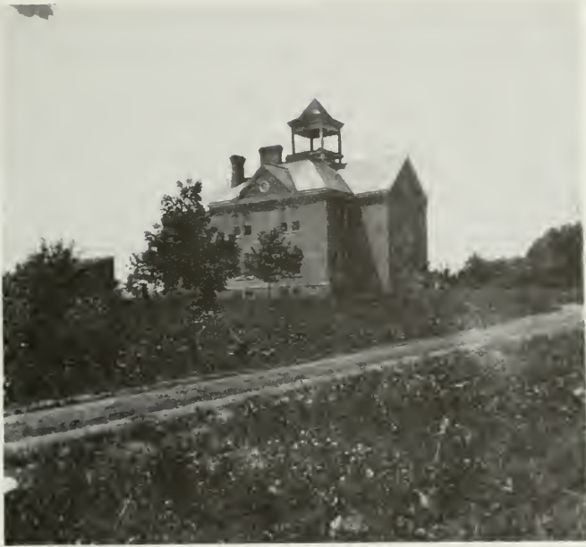
SOUTH SIDE [LOWE] SCHOOL
