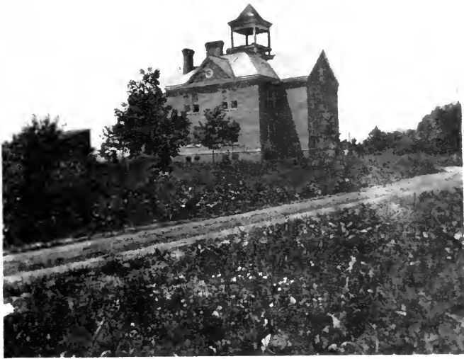
SOUTH SIDE [LOWE] SCHOOL
