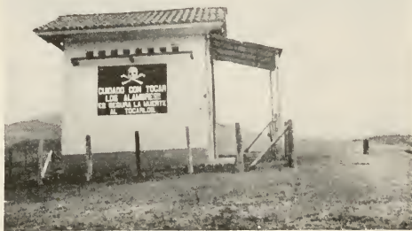
Skull and bones to warn the illiterate away from a high-tension electric station
