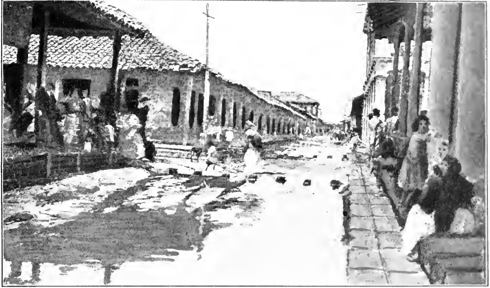
A STREET OF SANTA CRUZ DE LA SIERRA AFTER A SHOWER, SHOWING THE ATOQUINES OR PROJECTING SPILLES BY WHICH PEDESTRIANS CROSS FROM ONE ROOFED SIDEWALK TO ANOTHER
