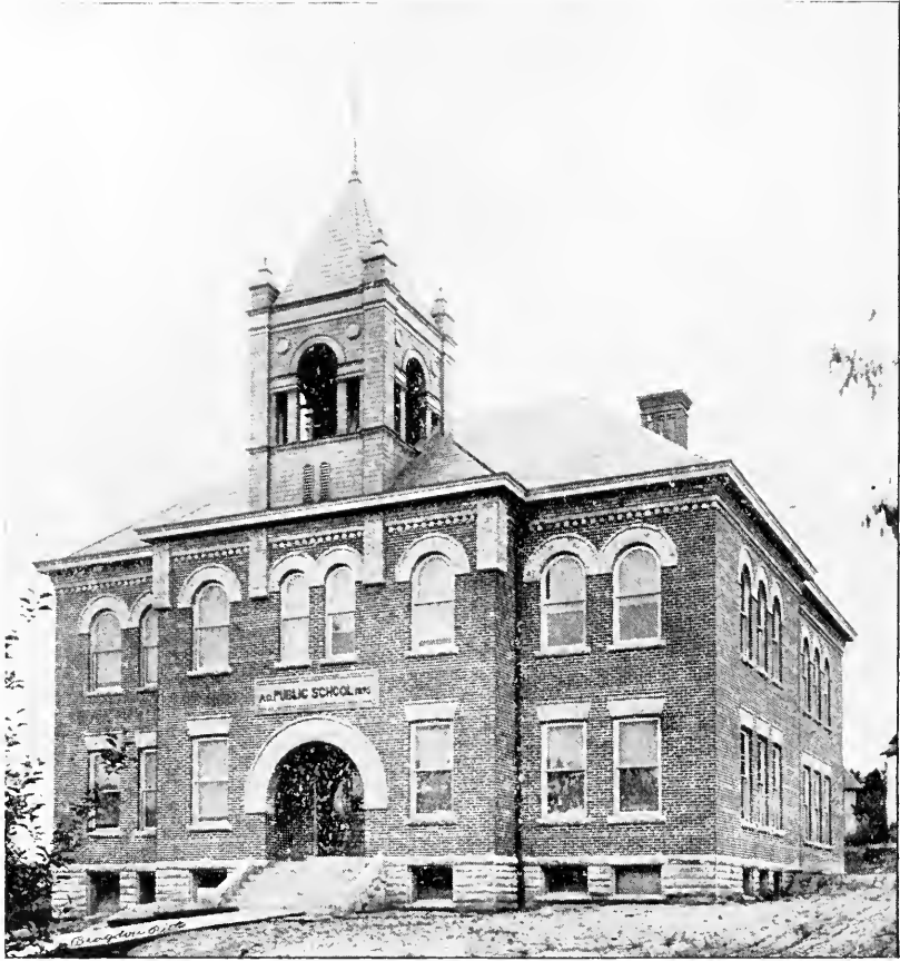
The Fourth School Building.
