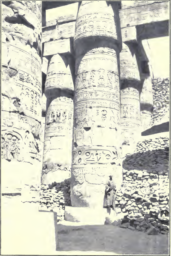
14. KARNAK, COLUMNS OF THE SIDEL-AISLI, HYPOSTYLE HALL.
