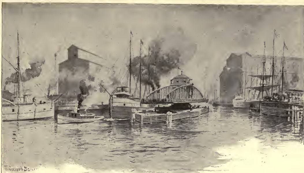
A STREET BRIDGE ACROSS THE CHICAGO RIVER, SWUNG OPEN FOR THE PASSAGE OF BOATS.
