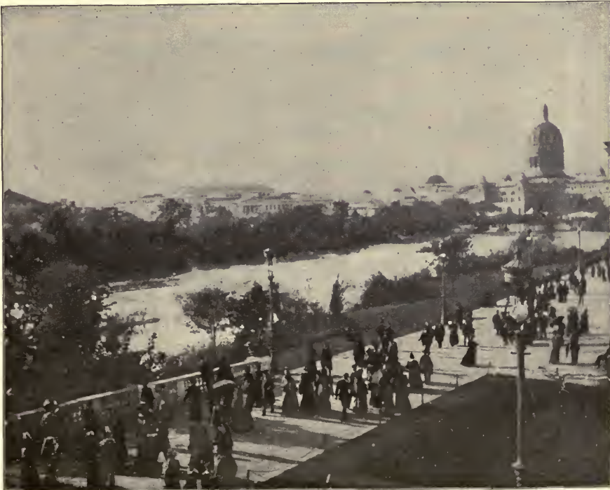
FROM A WINDOW IN THE MANUFACTURES AND LIBERAL ARTS BUILDING LOOKING NORTHWEST.
