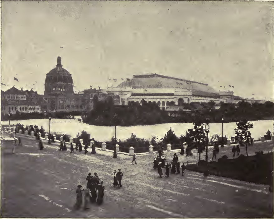
ANOTHER VIEW OF THE MANUFACTURES AND LIBERAL ARTS BUILDING.
