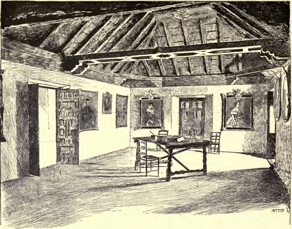
CELL OF THE PRIOR MARCHENA IN THE ORIGINAL CONVENT,—THE "COLUMBUS ROOM" IN THE MODEL AT THE FAIR.
