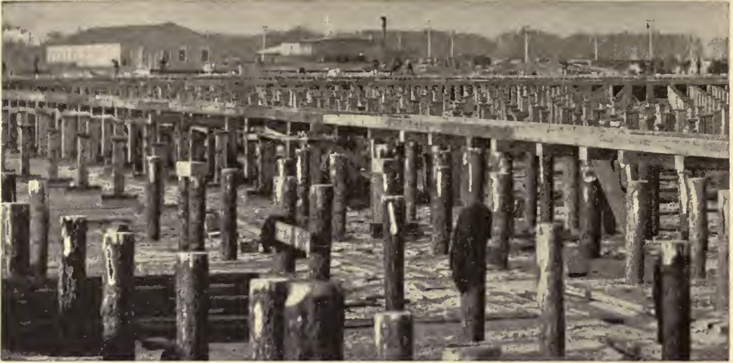
THE FOUNDATION OF THE MANUFACTURES
