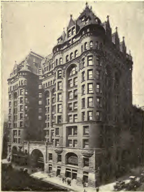
THE WOMAN'S TEMPLE. LA SALLE AND MONROE STREETS. (From a photograph by J. W. Taylor.)
