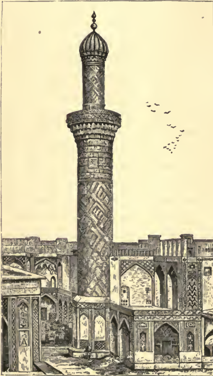
Fig. 142.—Shrine of Imam Hussein, at Kerbela. Showing the Use of Tiles in Persian Architecture.
