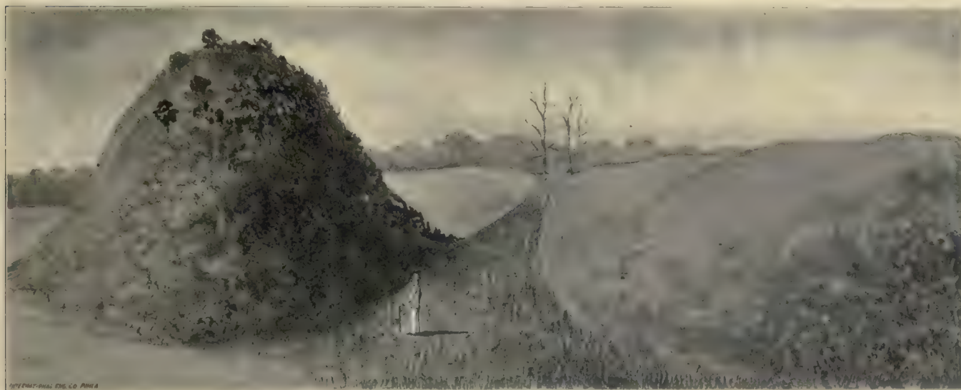
FIG. 7.—Principal mound with portion of main canal. Mound Island.
