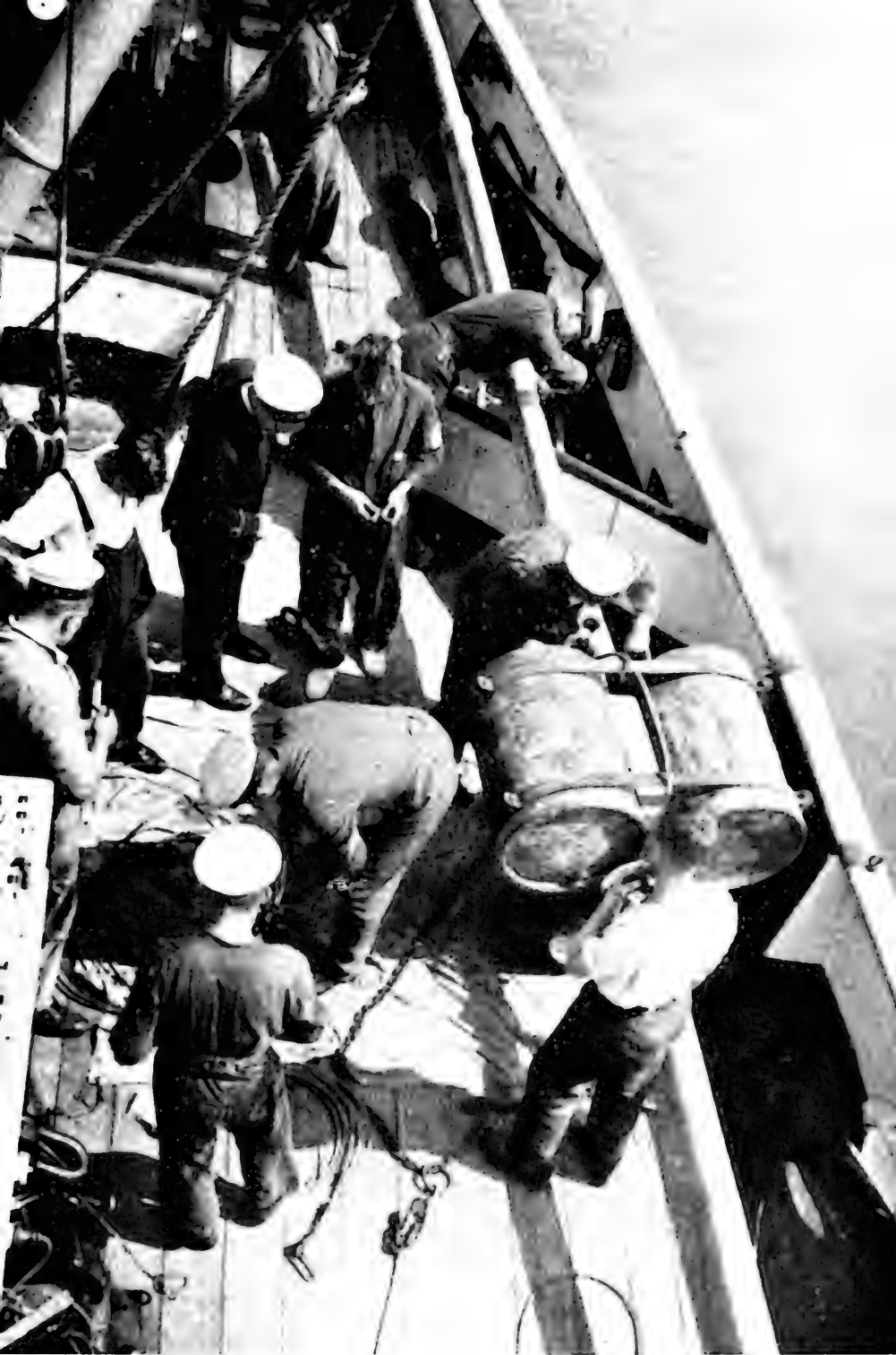
RIGGING A SURVEY BEACON ON DECK
