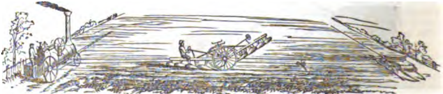
Fig. 12.—Fowler's Anchor, Engine, and Plough at work.
