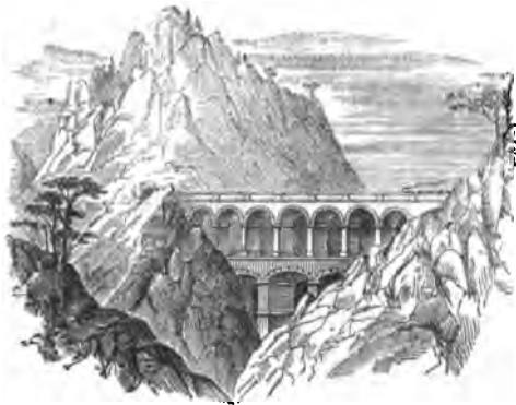
The Bollerswand Viaduct on the Great Sömmering Railway.
