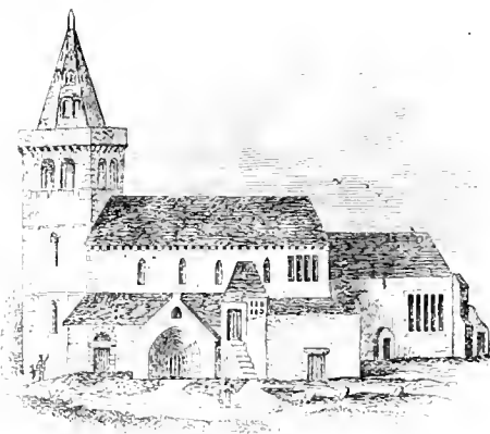
Crail Church (before the restoration).
