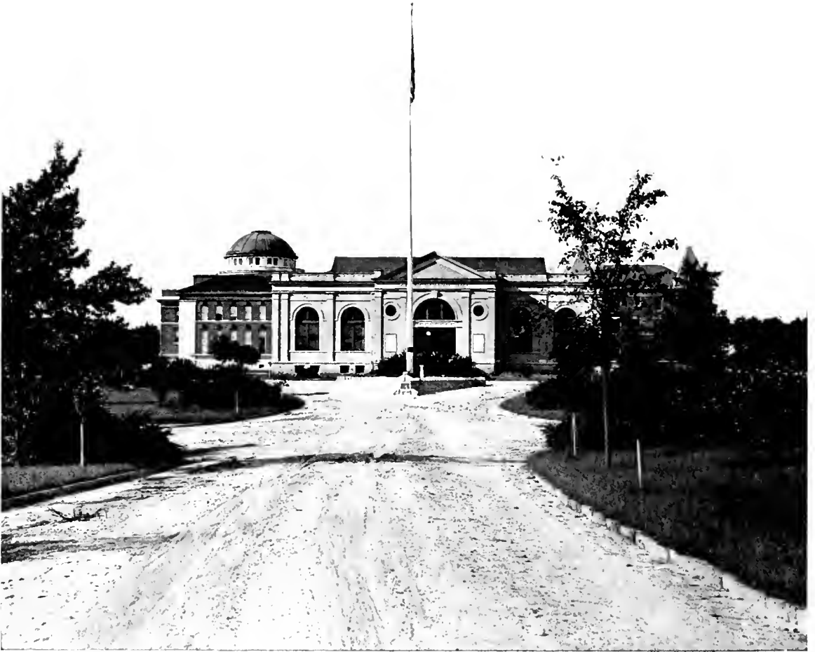
DRIVEWAY TO MEMORIAL HALL
