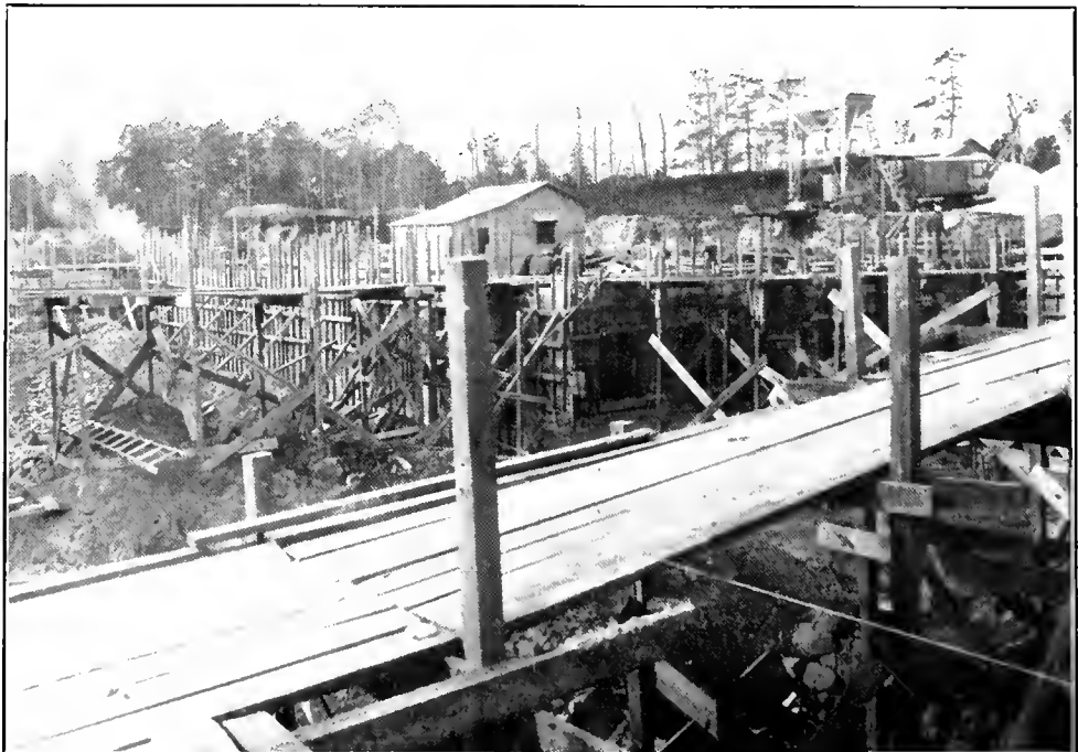
MEDICAL SCHOOL FOUNDATIONS BEING SET
