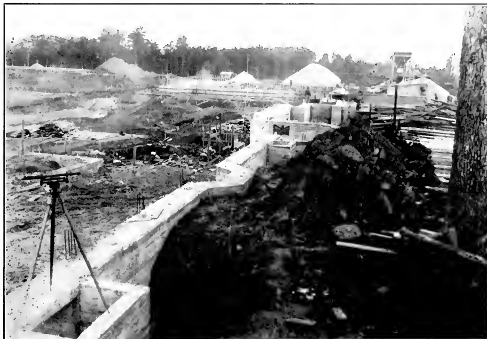
FOUNDATIONS FOR GROUP "C" DORMITORIES
