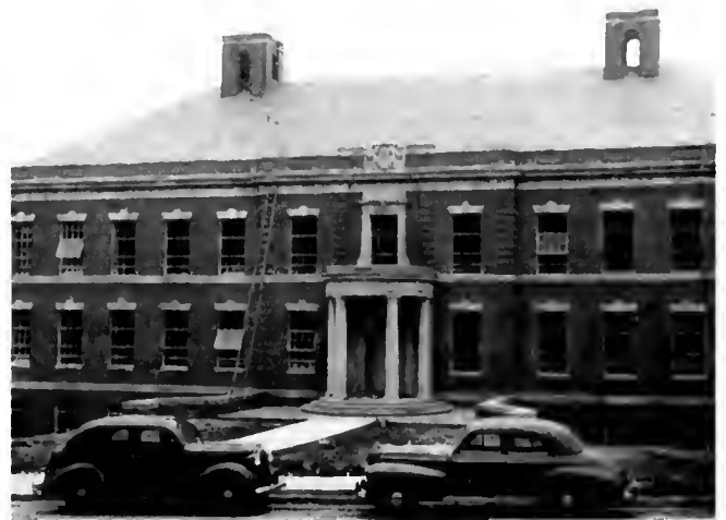
The Engineers have moved completely to West. Classes were held in their new building beginning the second semester of this year.
