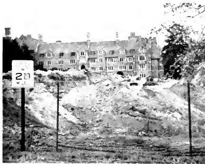
The construction of another new dorm . . .
