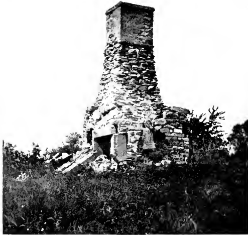
CHIMNEY OF THE HOUSE WHERE BENJAMIN PALMER WAS BORN.
