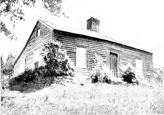
THE DART HOMESTEAD, SOUTH GLASTONBURY.
