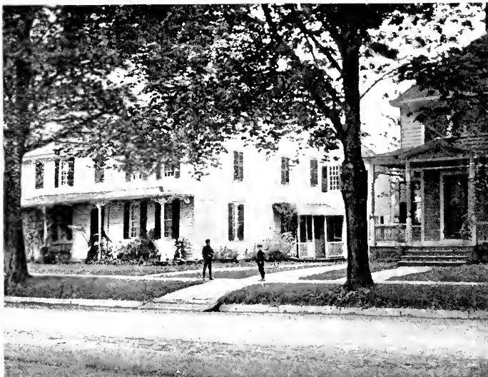
THE HOME OF ISRAEL KIMBERLY AND THE BIRTHPLACE OF EZRA KIMBERLY, PATRIOT, WEST HAVEN.
