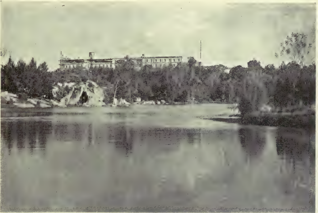
View of the Castle, from one of the lakes.
