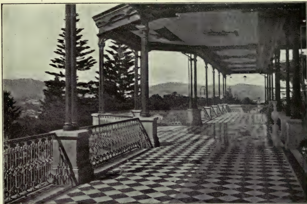
A terrace at the North wing.
