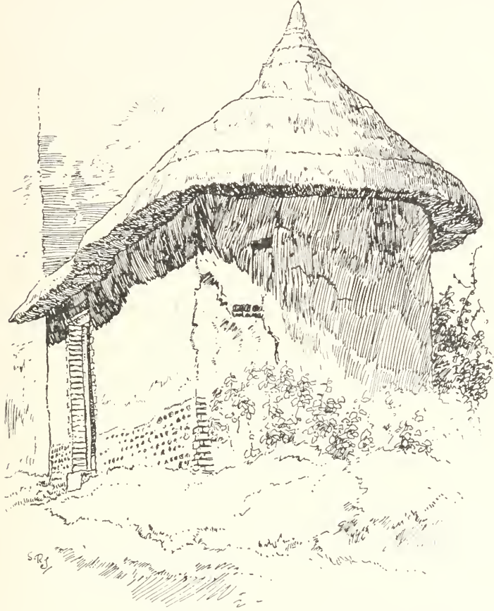
THATCHING AT CODFORD ST. PETER, WILTSHIRE
