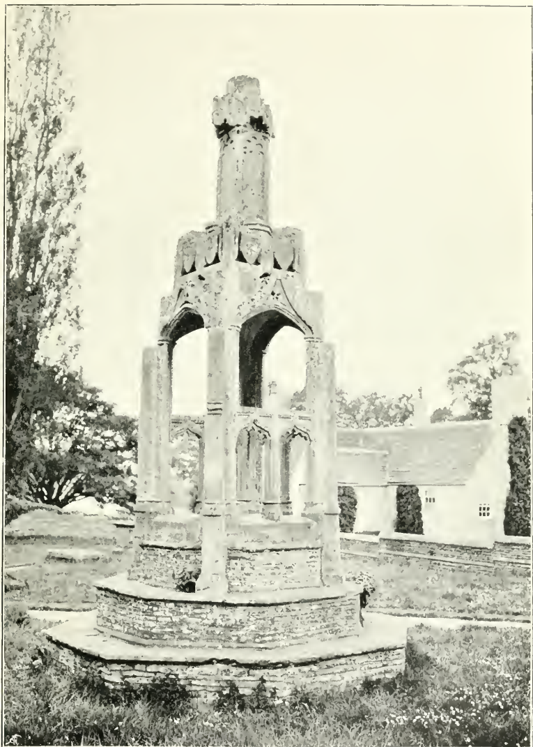
DECAYED PREACHING-CROSS IN IRON ACTON CHURCHYARD.
