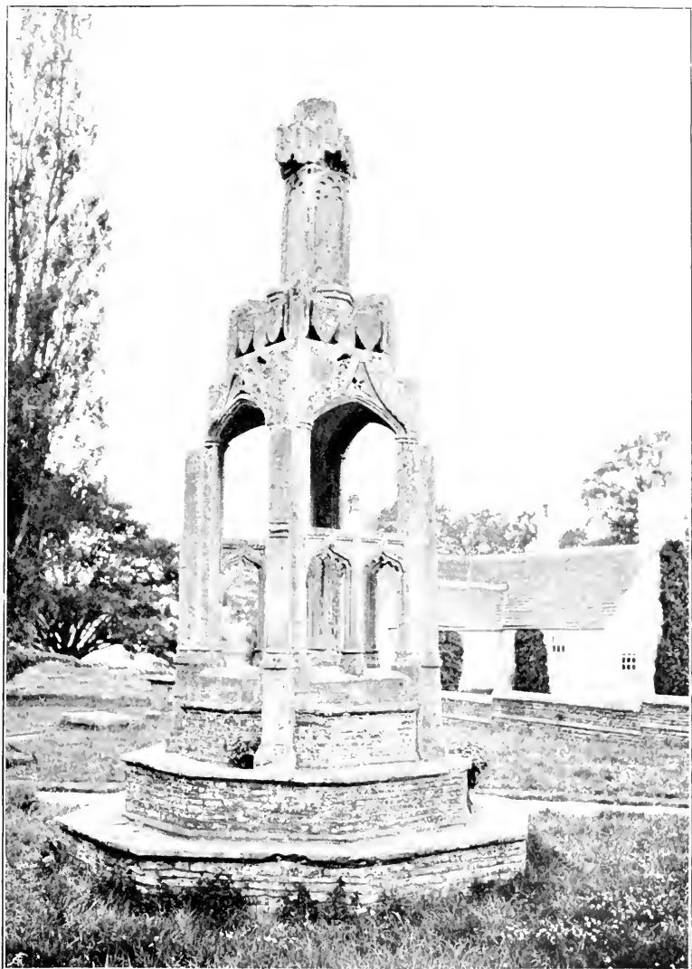
DECAYED PREACHING-CROSS IN IRON ACTON CHURCHYARD.
