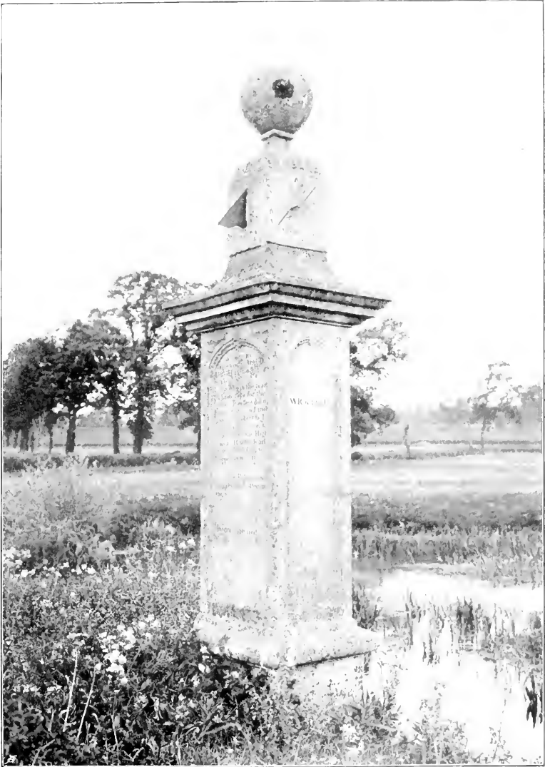
MAUD HEATH'S PILLAR, NEAR CHIPPEXHAM.
