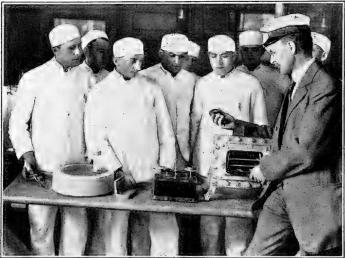
Fig. 18A.—Students Using Cheese Moisture Test.
