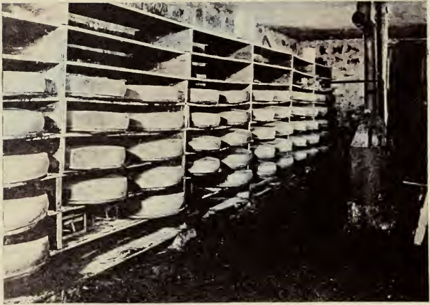
Curing cellar in Five Corners factory, near Monroe. The large drum Swiss cheese are on the shelves. The small boiler supplies steam for moisture when too dry.
