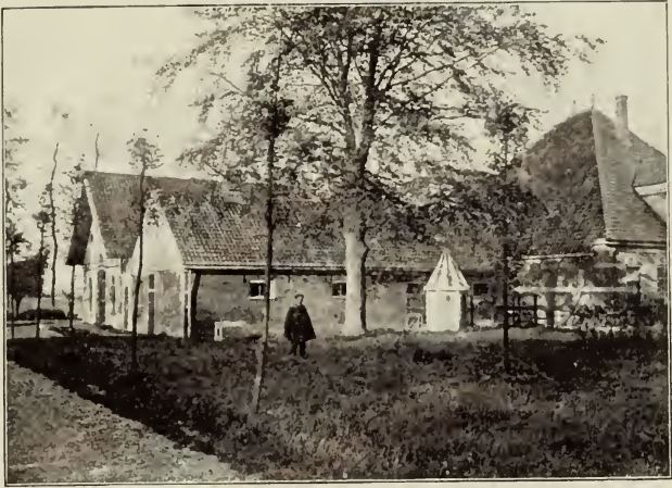
Farm buildings at De Rijp, North Holland.
