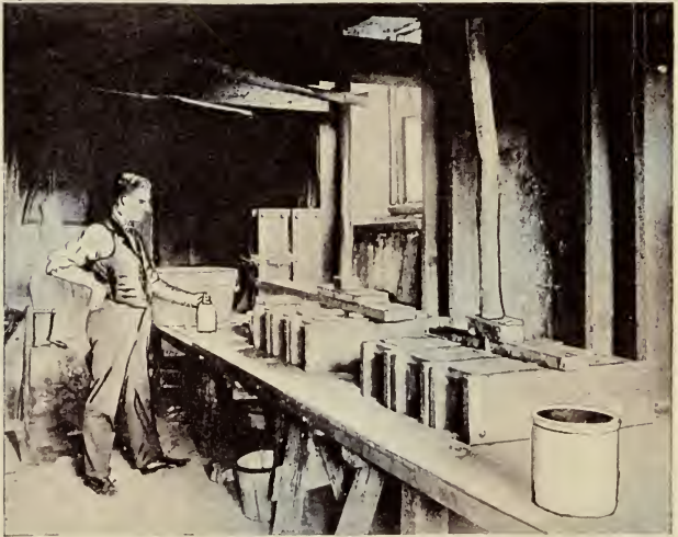
Block Swiss under pressure in individual molds.
