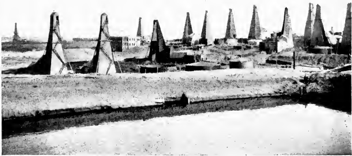
FIG. 82.—BINAGADI NEAR BAKU, CASPIAN. AMBAR OR EARTH STORAGE RESERVOIR CONTAINING CRUDE OIL IN FOREGROUND.
