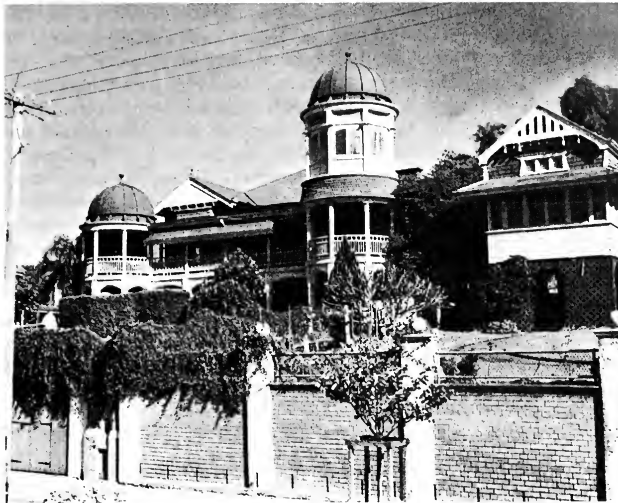
ANNEX BUILDING, CHEMICAL WARFARE SCHOOL, BRISBANE, AUSTRALIA
