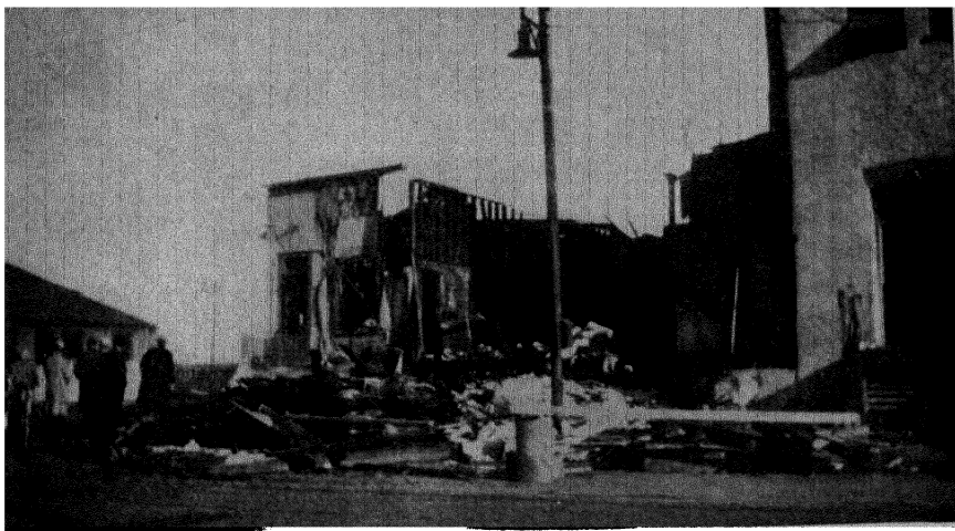
FIG. 36-9.—A flour-dust explosion at Omaha, Nebraska, caused this disaster.
