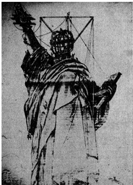
FIG. 27-9. — This rare old photograph shows the operation of putting the copper garment on the Statue of Liberty.
