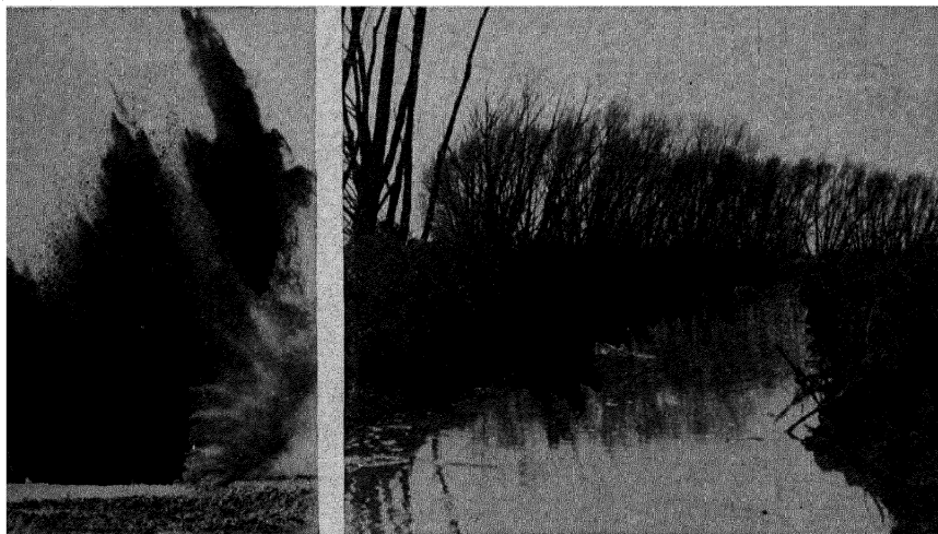
FIG. 6-10.—One chemical change makes way for others. The pictures show a drainage ditch being blasted and the ditch after the blast.
