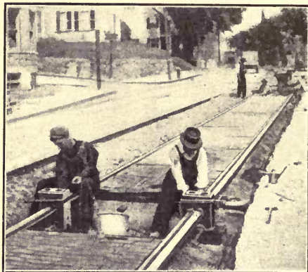
FIG. 123. — Thermit welding. Preparing molds about rail joints.
