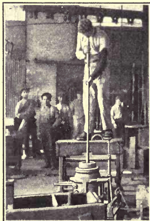
(b) Blowing a bottle in a mold.
