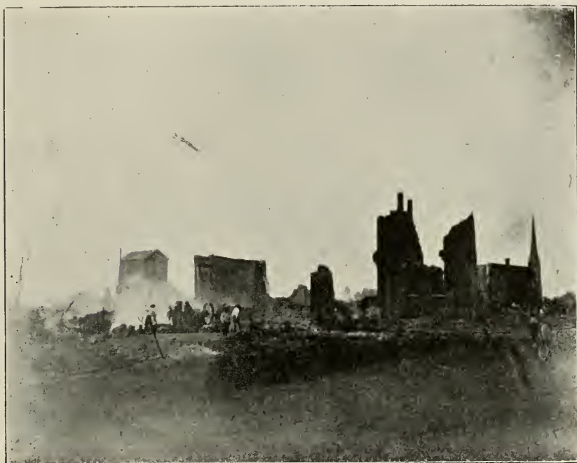
FIRE RUINS — LOOKING FROM EAST TO WEST
