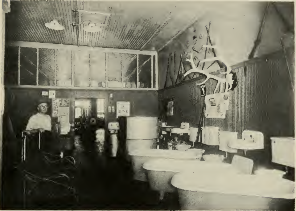
L. M. WILSON'S PLUMBING SHOP
