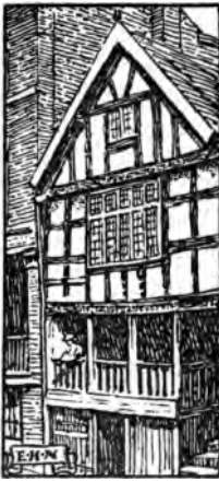
GOD'S PROVIDENCE HOUSE BEFORE RECONSTRUCTION
