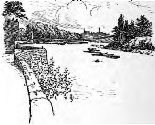
RIVER AND SUSPENSION BRIDGE
