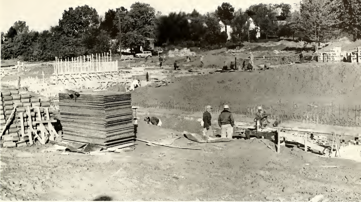
Planning an extensive building program, one of the structures started early in the year was the Training school.
