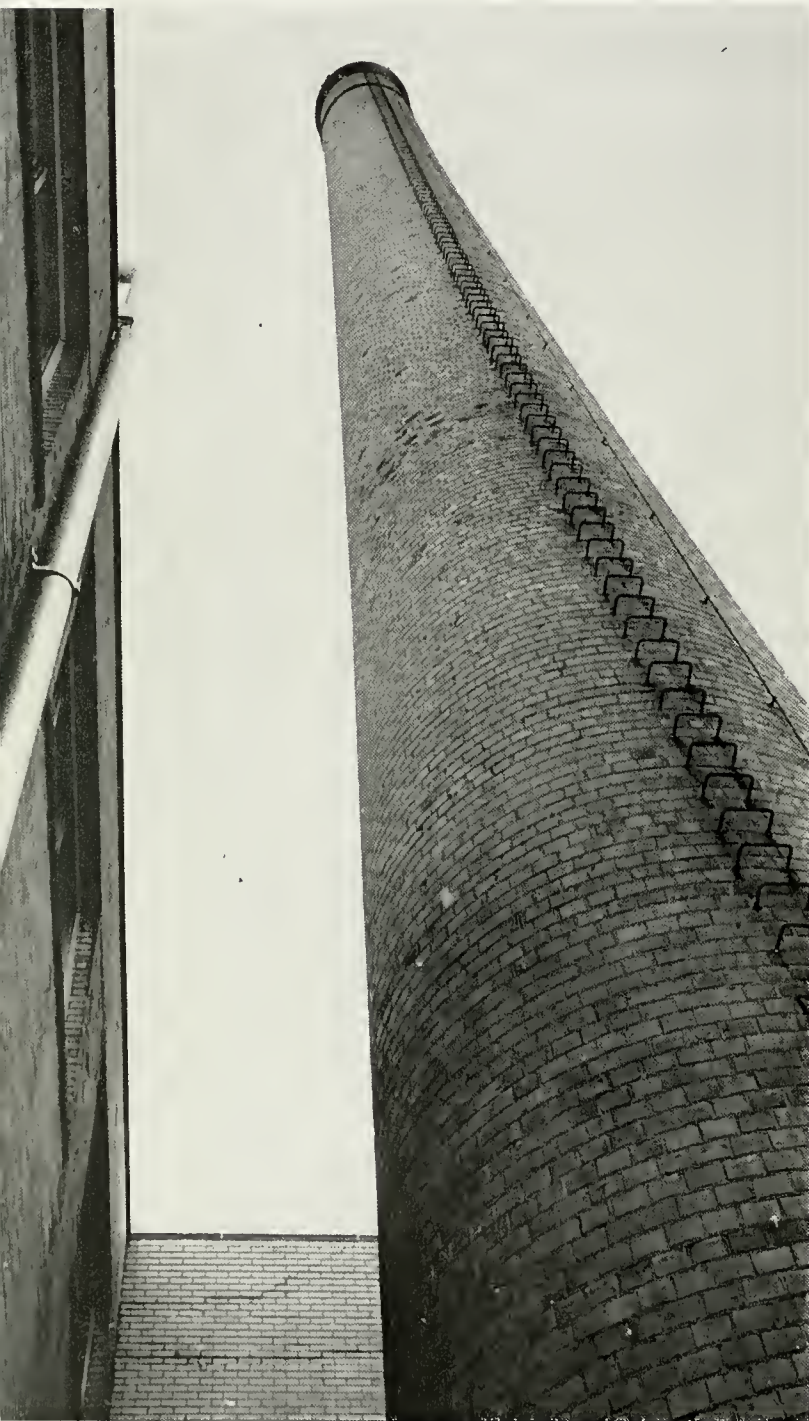
The physical plant as represented by the smoke stack of the heating plant is where the transfer of knowledge takes place.
