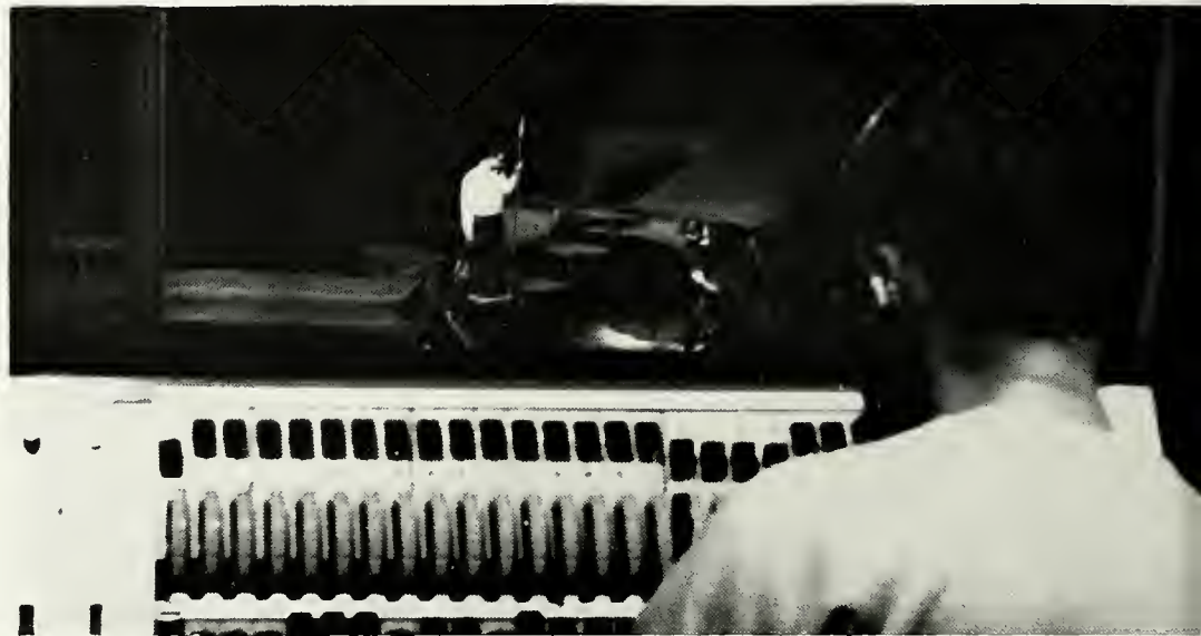
A glassed-in control room behind the audience houses the master unit which governs stage lighting.
