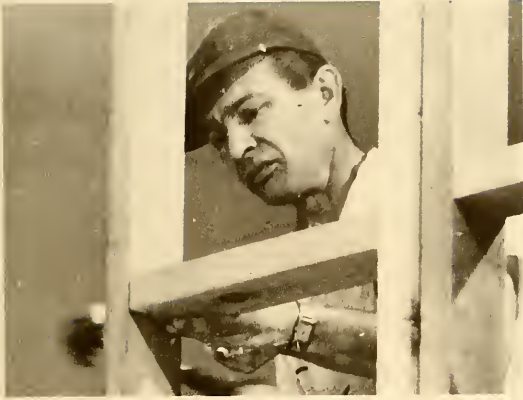
WORKMAN'S CONTRIBUTION Nailing a firm foundation.
