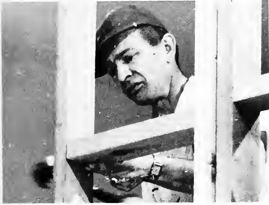
WORKMAN'S CONTRIBUTION Nailing a firm foundation.
