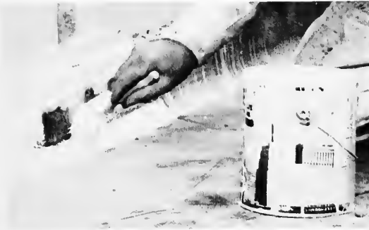
Painter Adding the final touch.
