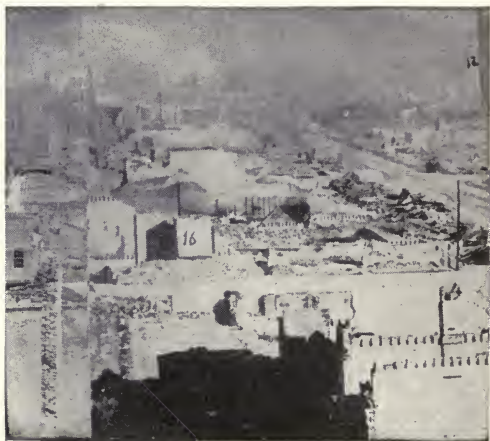
The Vault (No. 16), all that remained of Peacock's store after the Chicago fire in 1871
