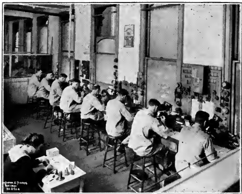
Section of Polishing Room
