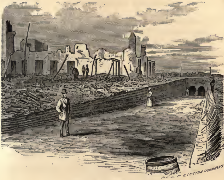
LASALLE STREET TUNNEL.
