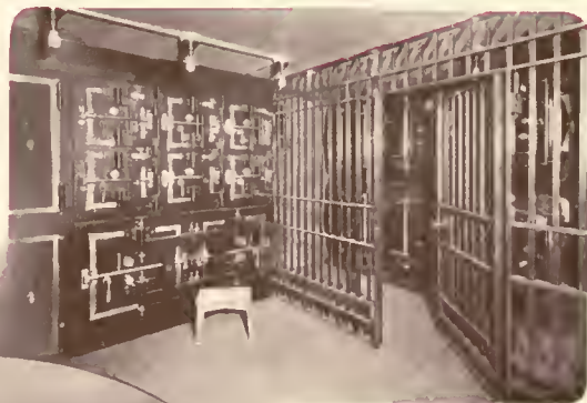
Cash Vault of Bank
