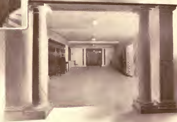
Lobby of Safe Deposit Vaults
