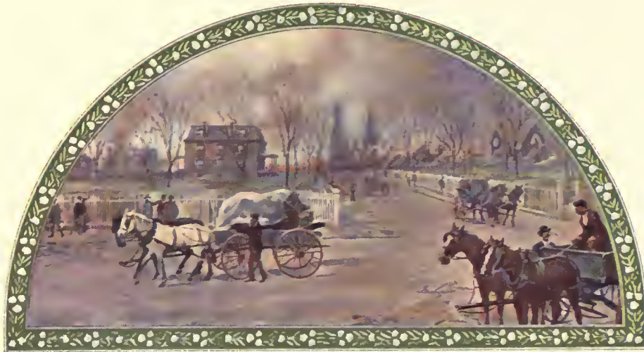
OGDEN HOUSE AFTER THE FIRE
