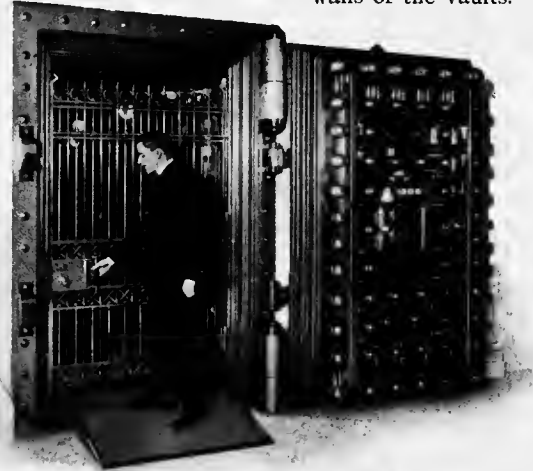
Entrance to Vault
