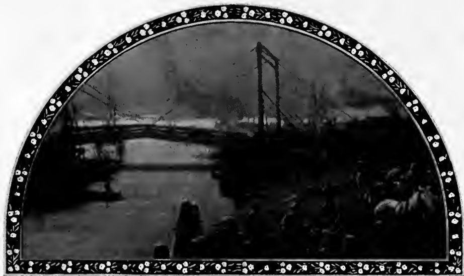
DEARBORN STREET BRIDGE
