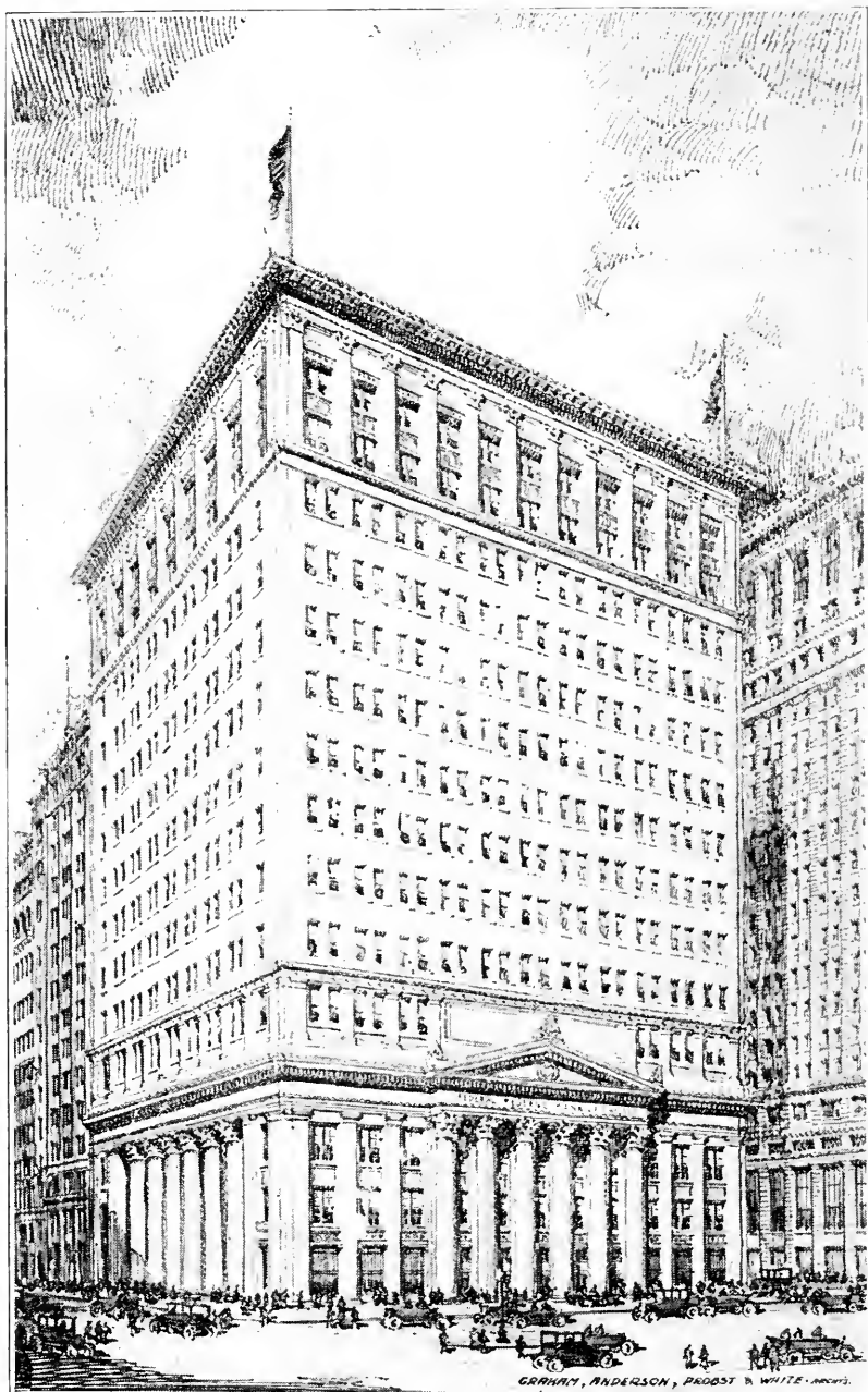
Federal Reserve Bank of Chicago, now under construction.
