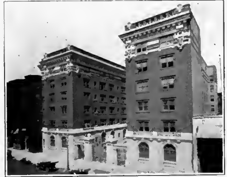
ST. LUKE'S HOSPITAL
