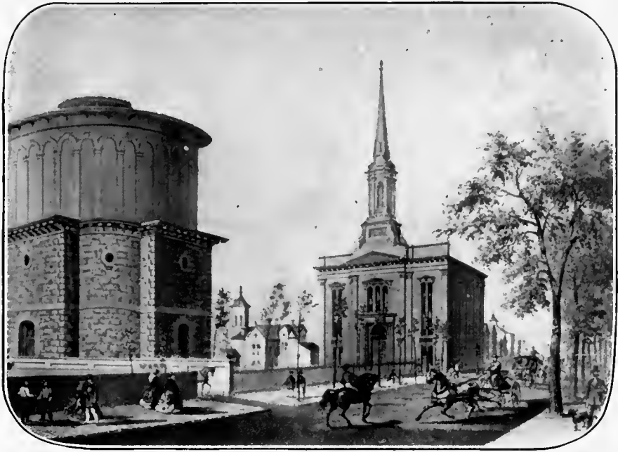
WATER RESERVOIR AT THE CORNER OF MORGAN AND WEST MONROE STREETS
