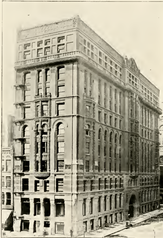
PHENIX INSURANCE BUILDING. Supplied with Hale Elevators.
