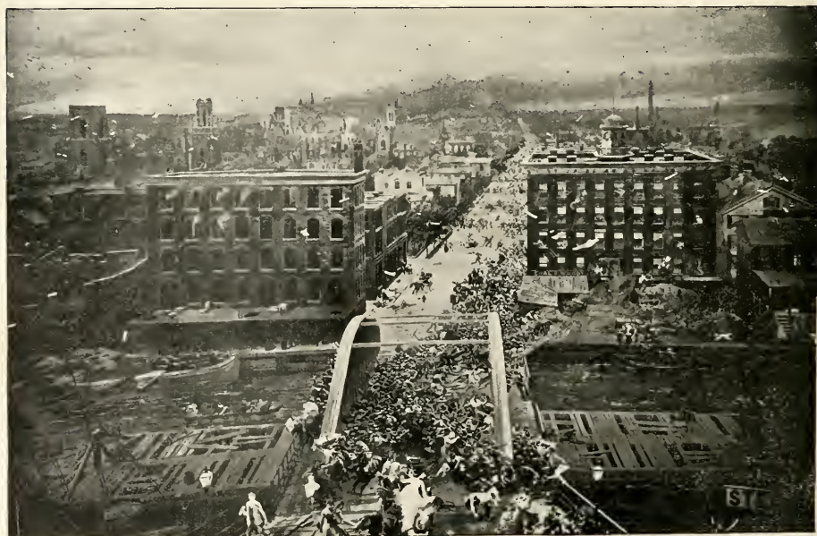
RUSH STREET BRIDGE, LOOKING NORTH.
