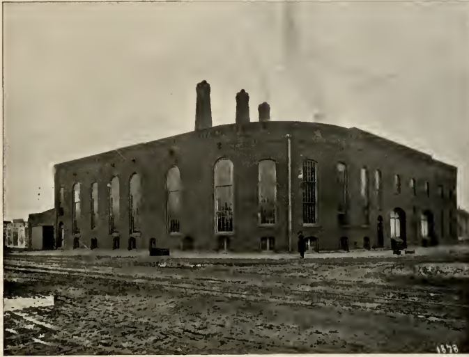
POWER HOUSE, CHICAGO CITY R. R., COTTAGE GROVE AVE AND 55TH STREET.
