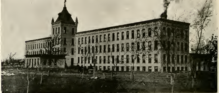
C. M. HENDERSON & CO'S. NEW FACTORY AT DIXON ILLS. CAPACITY 5000 PAIRS DAILY.
