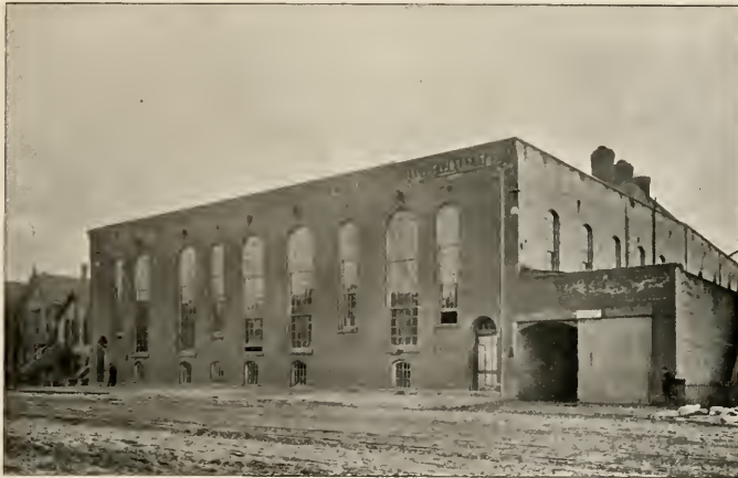
POWER HOUSE, CHICAGO CITY R. R., STATE AND 53RD STREET.
