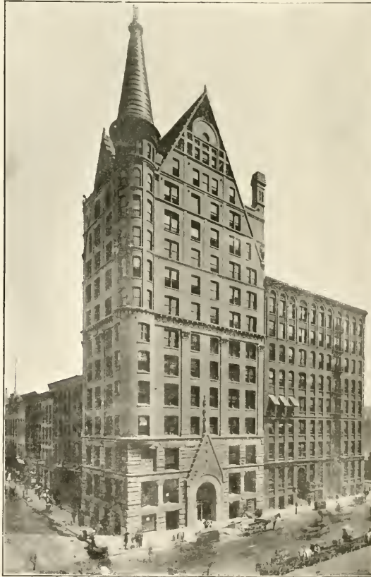
OWINGS BUILDING, HEADQUARTERS OF LOBBELL, FARWELL & CO. Supplied with Itale Elevators.
